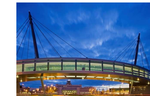
>Dublin Airport, Pier D Terminal
